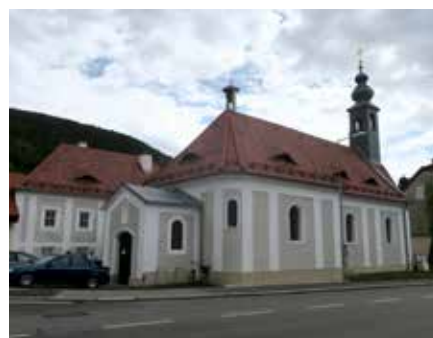
Fig. 92 St. Helena Church in Helenen Valley; was restored in 2018, financed by the catholic parish and private donators (about 60%) as well as subsidies from the City, Province and Federal Monument Authority.
