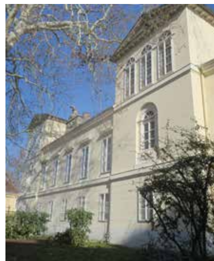
Fig. 89 Florastoeckl; Part of the Federal High School; 1827 to 1830 residence of crown prince Ferdinand.
